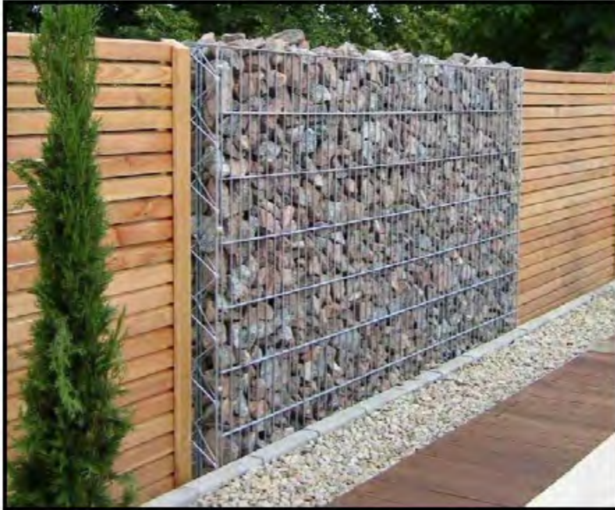
Figure 9 - Proposed 6' Gabion/Wood Fence
